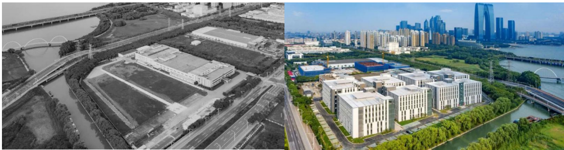
Figure 6: Before and after renovation of Xinhong Industrial Park.
