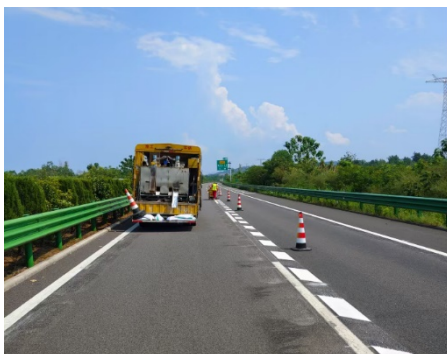
Figure 1: Laying on the Downhill Section Edge Rate Marking Line.
