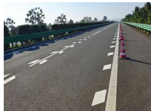
Figure 1: Laying on the Downhill Section Edge Rate Marking Line.
