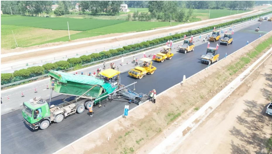
Figure 1: Construction Site of Highway Reconstruction and Expansion Project.
